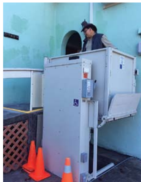
Pastor David Moon-Wainwright operates a new wheelchair lift installed at the back door of the church.
