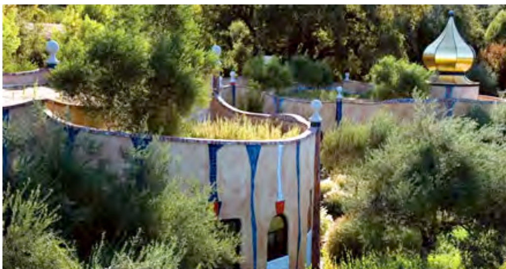
In Napa's Stags Leap District, Quixote winery conserves energy and reduces water run-off with a sod roof planted with trees and shrubs to blend into its surroundings.
