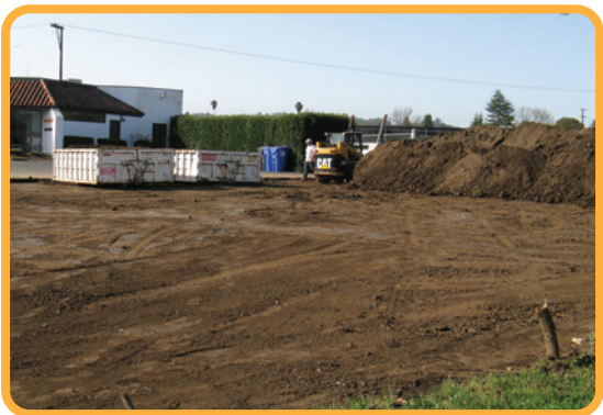
The work in progress
