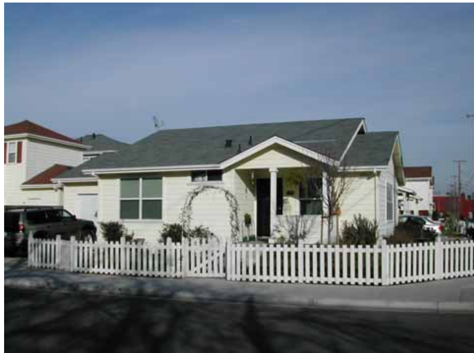
Deturk self-help housing developed by Burbank Housing provided new homes for 32 families in a convenient downtown Santa Rosa location.
