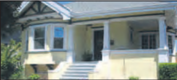
Gorgeous Victorian Home with original detailing-lead glass windows, coved ceilings, built-in china cabinet, 2-car detached garage and full basement w/3 add'l bedrooms & bath. 1400DB $699,000 3 bdrm/1 bath Napa
