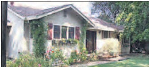
Wonderful Home on a Great Street with a detached studio and a detached office building on over half an acre of lawns and gardens. Room for a pool, bocce court or gentleman's vineyard. 1490CR $990,000 2 bdrm/2 bath Napa
