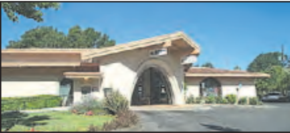
1400 Clay St., Ste 100 - FOR LEASE: 4,822 SF +/- Ground flr pro ofcs w/ pking, new price reduction, 14 priv ofcs, high end improvements: conf rm, kitchenette, rr, waiting/recp area, server rm, cubicle area. $2.40/SF/Mo NNN Office Napa
