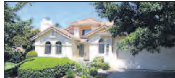
Silverado Country Club Home with tasteful designer touches throughout. The home features hardwood floors, plantation shutters, beautiful tile kitchen counter tops. Stunning archway entry. 1446KM $912,000 3 bdrm/2 bath Napa
